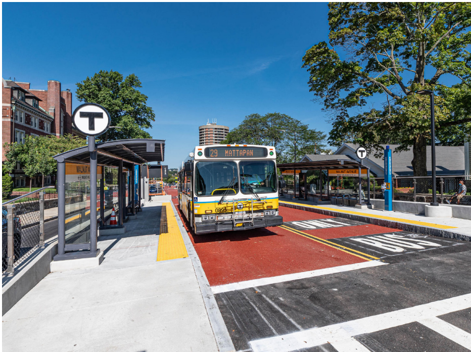
Figure 22: Bus lanes and bus stop on Columbus Ave
