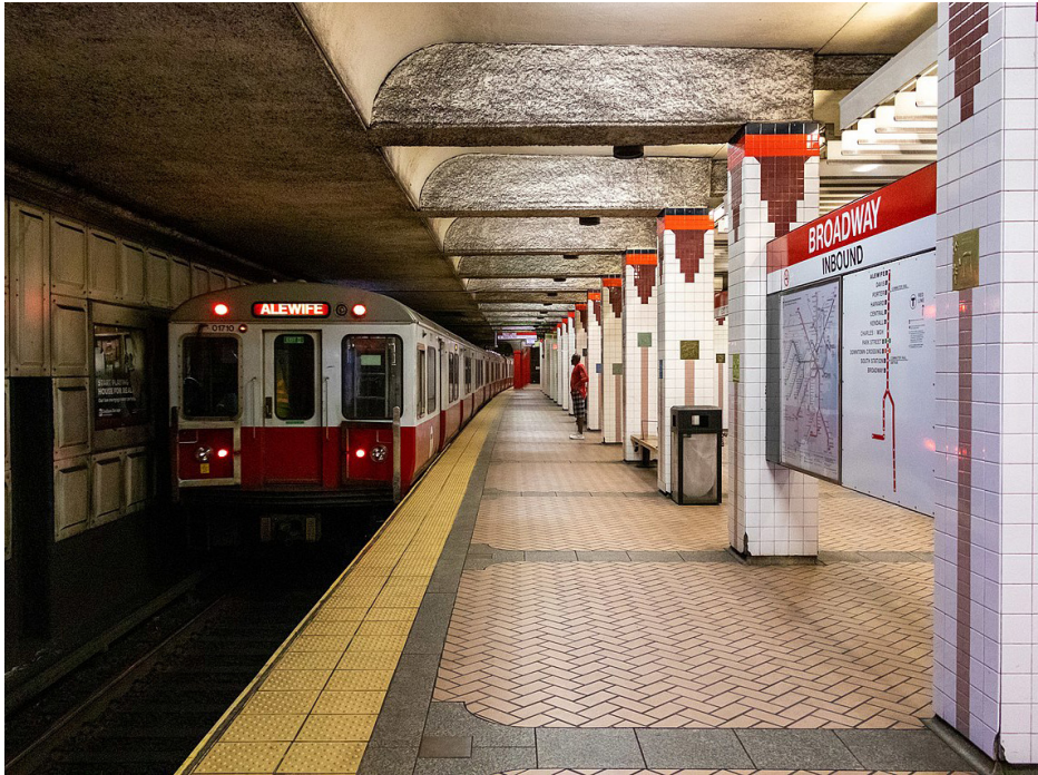
Figure 17: A Red Line subway train at a station platform
