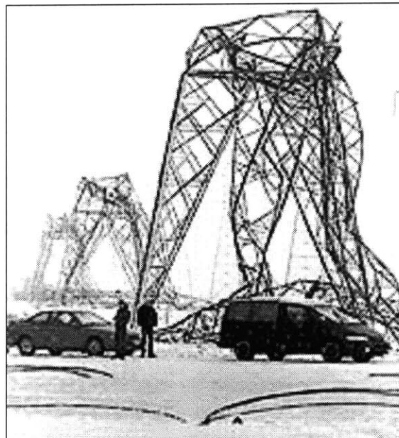
Figure 13.0 – Tower Damage, Quebec Ice Storm
