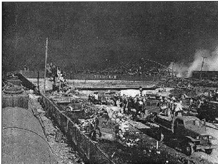
Figure 21.0 – 150-ft Barge Washed Ashore by Tidal Wave, TX City Disaster
