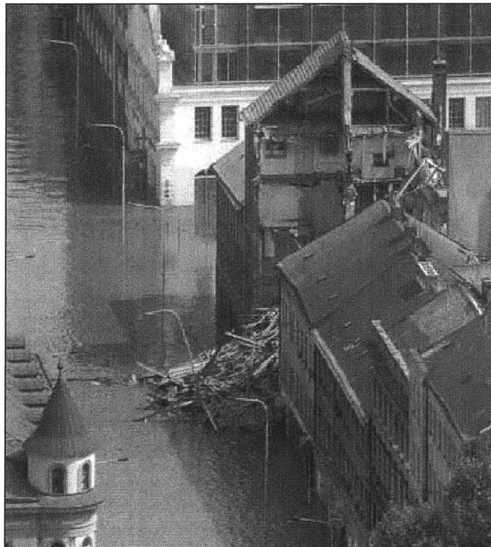
Figure 18.0 – Flood Damage in Prague, 2002
