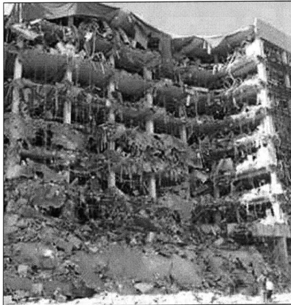
Figure 25.0 – Bomb Damage to Murrah Federal Building
