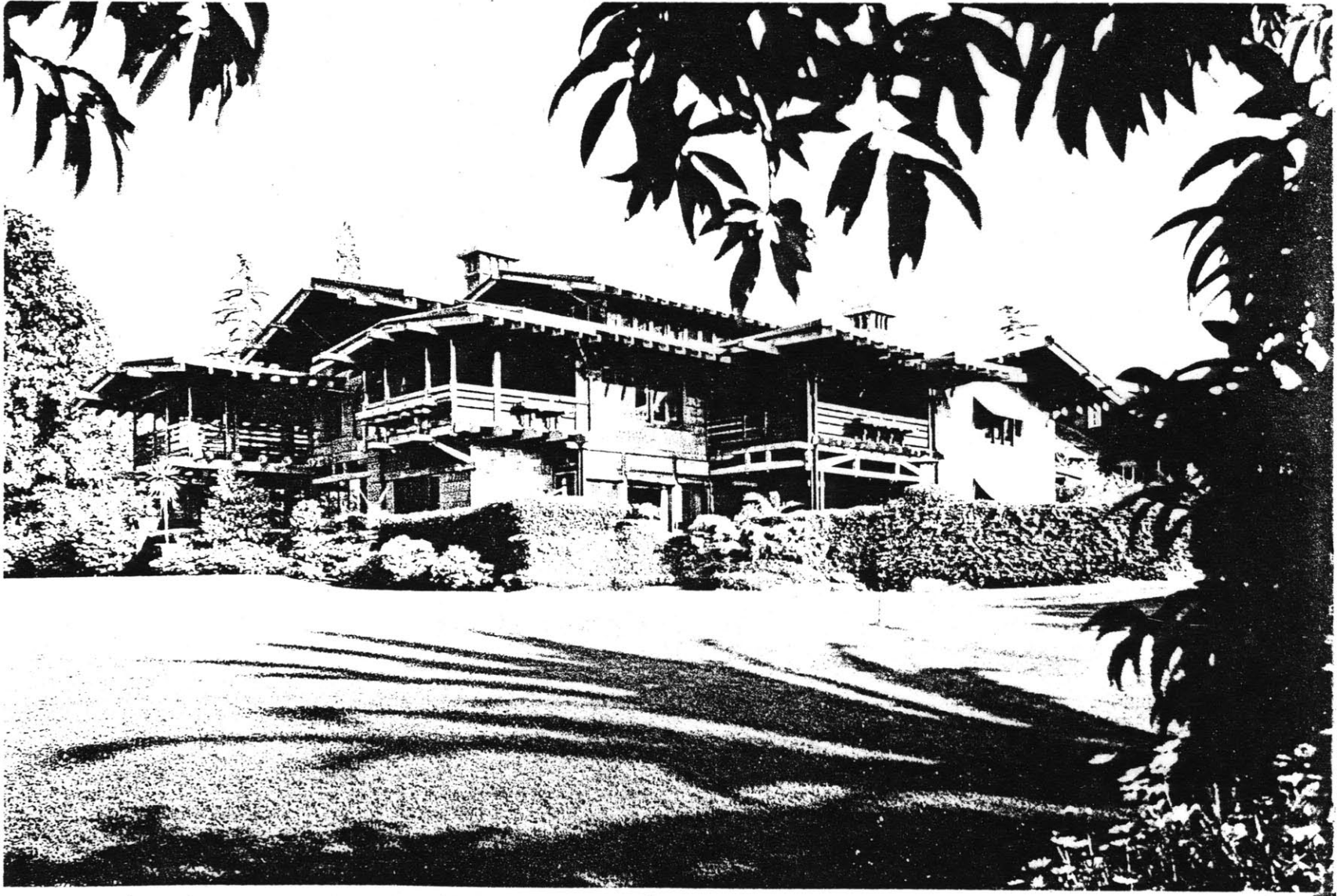
SWISS-JAPANESE STYLE LOGGIA/PAVILIONS. OPEN FRAMEWORKS AGAINST CONTINUOUS SURFACES. GAMBLE HOUSE BY GREENE + GREENE. SOURCE 41.
